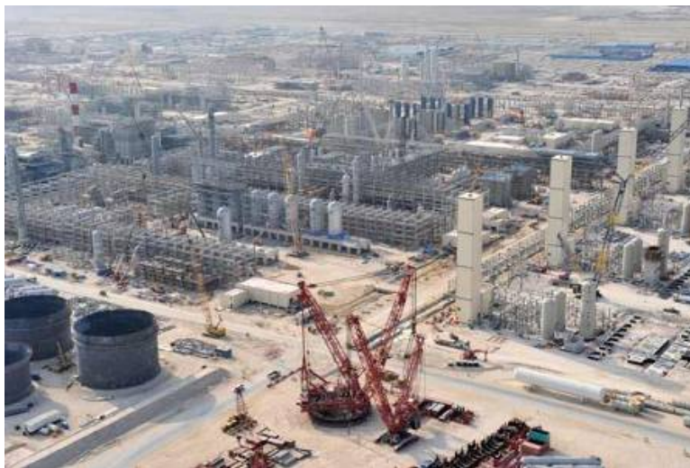
Figure 4-7: Qatar GTL Plant under Construction (Ref. /41/)
